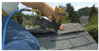
Install your ridge cap shingles according to shingle manufacturer's instructions. Remember to leave a 1" gap between the roof shingles and the cap shingle. When using a nail gun you should reduce the nail pressure so that you do not drive the nail home.
