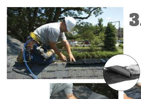
When the ridge length is greater than 20' or you are using leftovers from a previous job, you must create a joint to continue the vent. To join two pieces together, one piece must have a 9" flap and the other must be flush. Butt the four vent strips together and secure with caulk. Lap the 9" cap seal material over the joint using a bead of caulk under the lap to create a water-tight seal.
