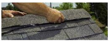
Mongoose Ridge Vent is designed to be used with different widths of ridge caps. If your ridge cap is smaller than total width of Mongoose (11"), trim excess cap seal on both sides of the ridge cap shingles.
