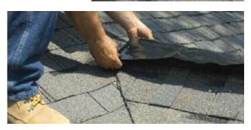
When finished applying Mongoose Ridge Vent, use the extra 9" cap seal material to create an end cap by folding the 9" flap under the vent material. (Mongoose Ridge Vent has 9" of extra material on both ends, it is important to tuck the extra 9" under both ends of the ridge – this creates end caps). Press Mongoose Ridge Vent to the roof, the glue will hold Mongoose Ridge Vent to the roof shingles.
